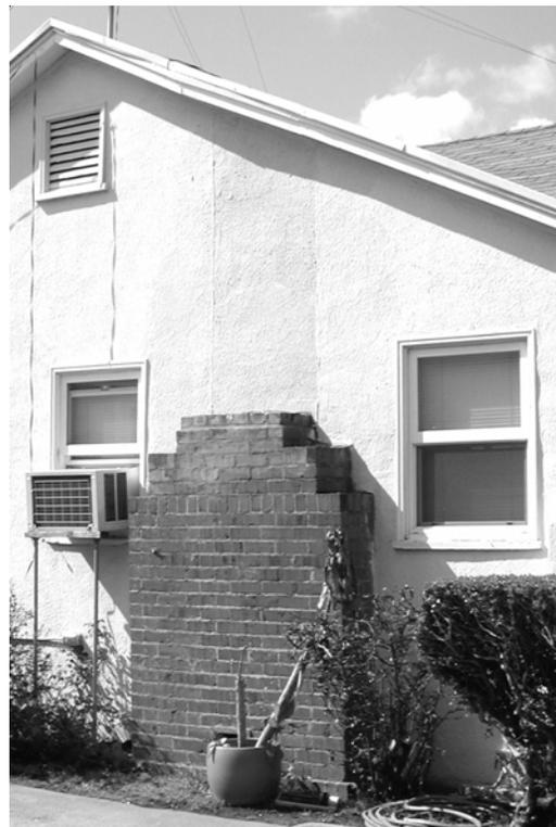
**Figure 35** - Photo showing damaged chimney removed. Note that the fireplace is now not functional.
